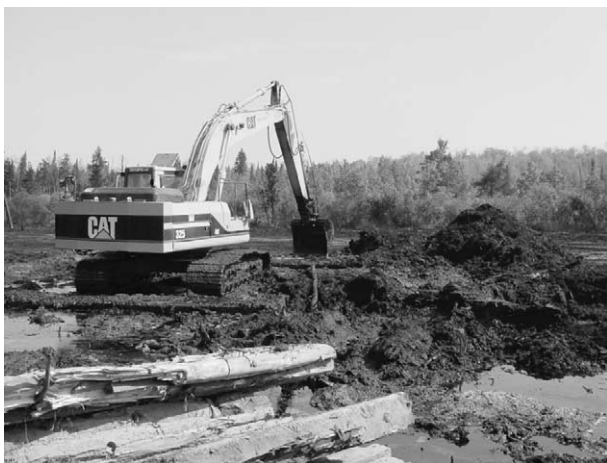
Fig. 2 A peat bog in Minnesota was burned to prevent crude oil from migrating into the nearby Mississippi River. Wooden mats needed to be placed on the bog to allow access by heavy equipment (photo courtesy State of Minnesota).
